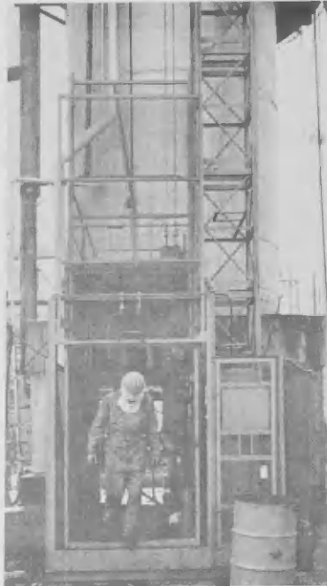
Here is the enclosure of the elevator at ground level. It is a portable level.
